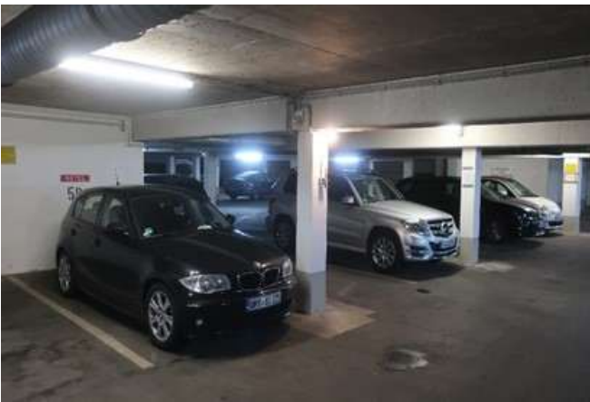
Underground parking area
