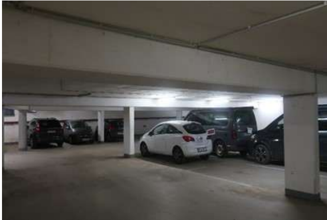
Underground parking area
