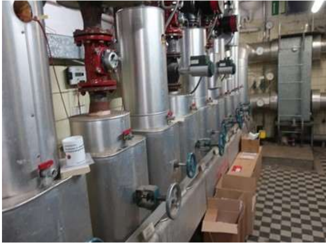
Building services, obsolete
