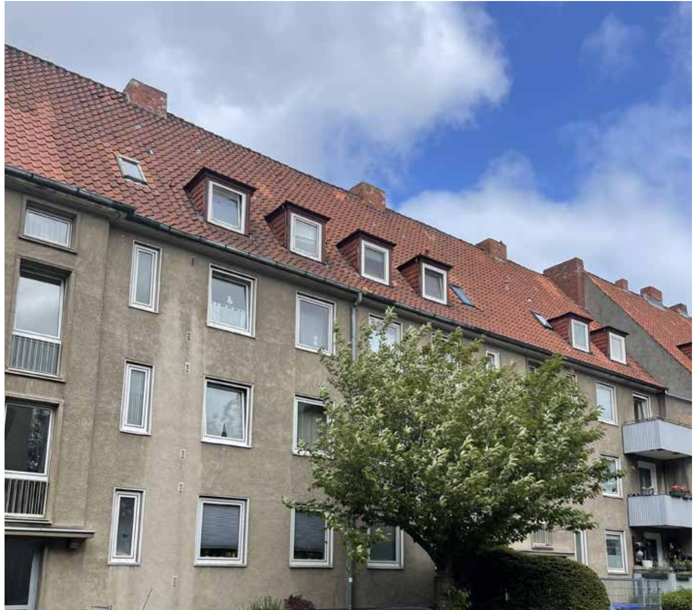
Georgstrasse, Lübeck for renovering.
