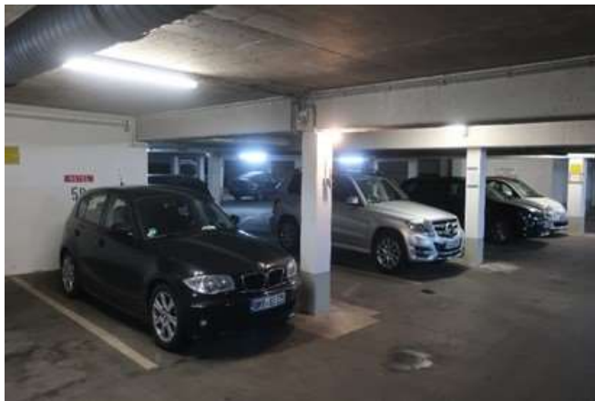
Underground parking area
