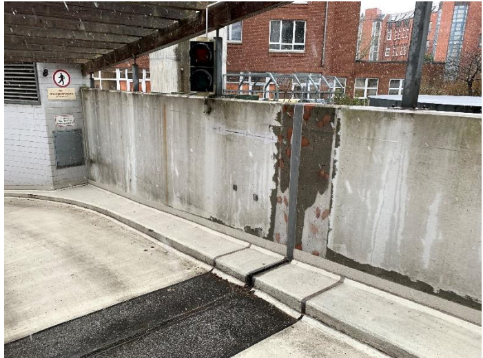
Repaired sealings, entrance underground parking
