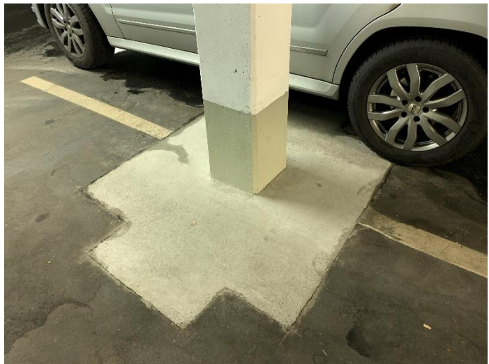
Repaired concrete damage in the underground parking
