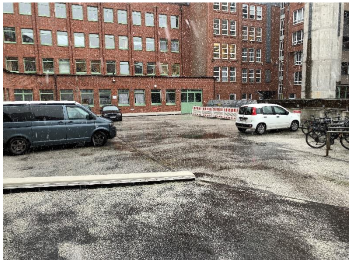
Renewed sealings and cover of yard area, underground parking roof
