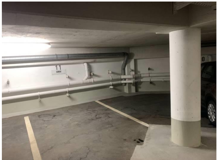
Plaster and concrete damage repaired in 2019
