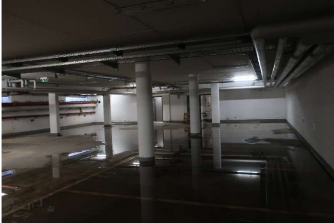
Underground parking area
