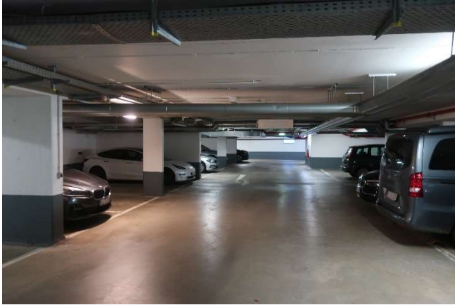
Underground parking area
