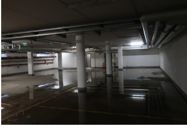
Underground parking area
